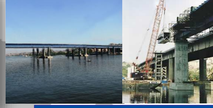
Izmit Bay Crossing Bridge (2016)
