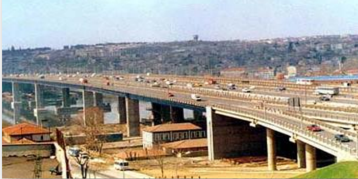
Old Golden Horn Bridge (1974)
