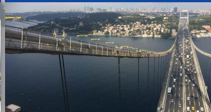
2nd Bosphorus Bridge Rehabilitation Project (2017)
