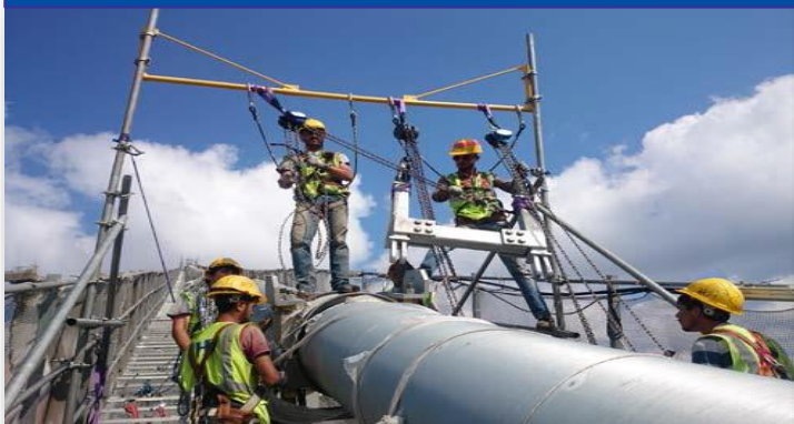
1st Bosphorus Bridge Rehabilitation Project (2019)
