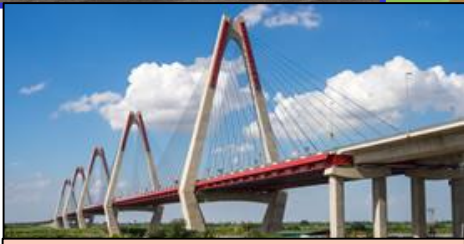
IHI Infrastructure Systems bridges
