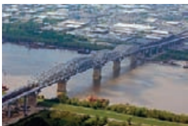
Huey P. Long Bridge in the U.S.
