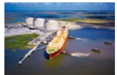
The Cameron LNG receiving terminal built for Sempra Energy (Louisiana, the United States)
