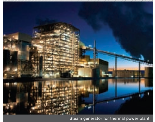
Steam generator for thermal power plant
