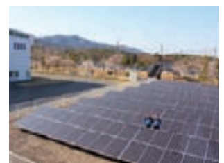
External view of solar power generation facility
