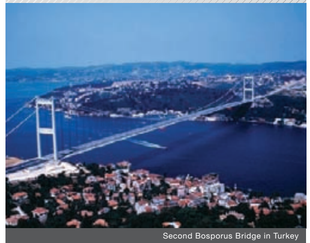
Second Bosphorus Bridge in Turkey
