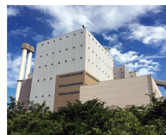
IHI delivered boilers to the No. 2 Thermal Power Plant in Kobe Steel's Kobe Works in 2004
