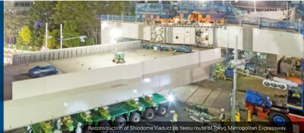
Reconstruction of Shiodome Viaduct on Yaesu route of Tokyo Metropolitan Expressway
