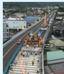
Bridge deck replacement work
