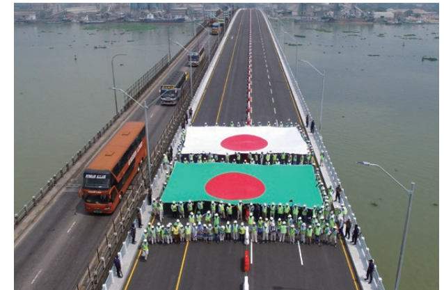
Completion of the new Meghna Bridge (existing bridge on left, new bridge on right)
