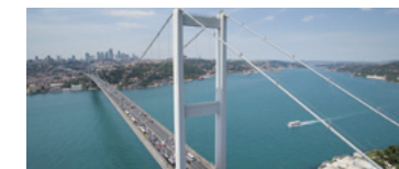
First Bosphorus Bridge after repair work
