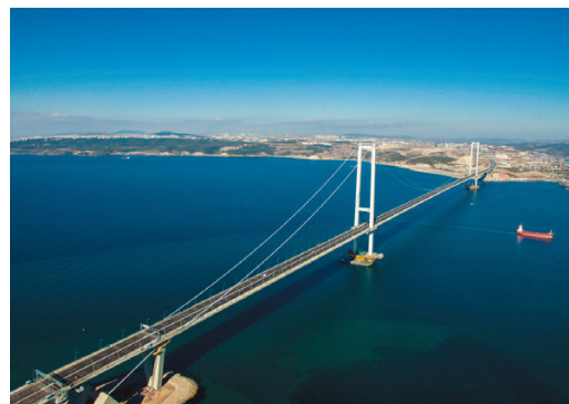
Izmit Bay Crossing Bridge
