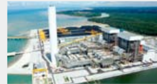
Jimah coal-fired thermal power plant in Malaysia, a previous project of IHI together with Sumitomo Corporation and Toshiba Corporation
