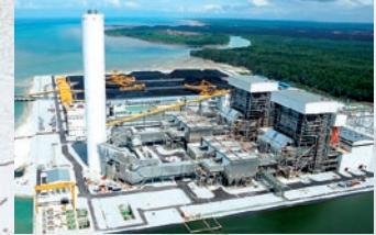
Existing Jimah coal-fired thermal power plant adjacent to the new power plant project site
