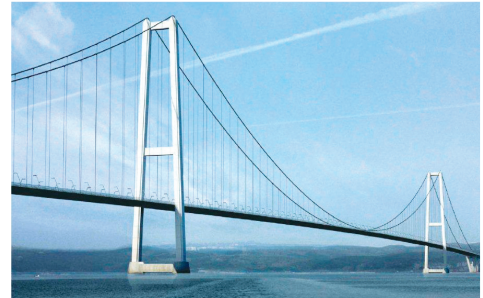
CGI representation of the completed Izmit Bay Bridge
