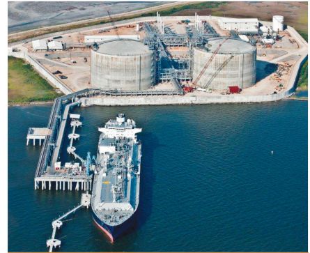
LNG receiving terminal handed over to Gulf LNG Energy LLC
