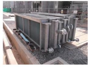
Inlet-air heating coil using steam
