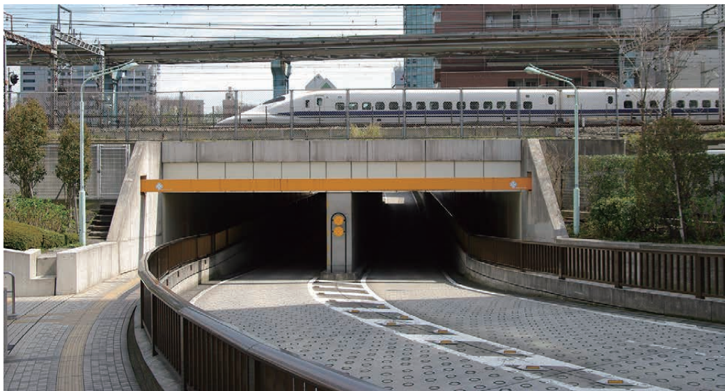
Grade separated railroad/road crossing constructed using the URT method
