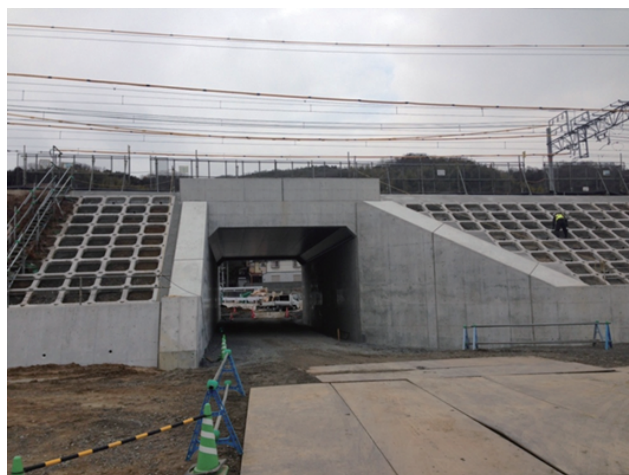
URT work without box beams for tension work at completion
