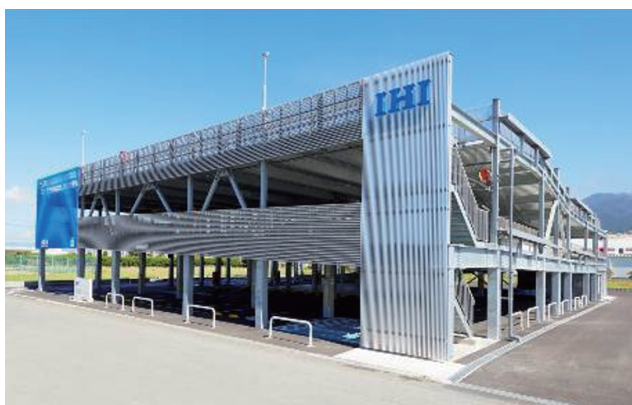
Demonstration test parking lot in Numazu
