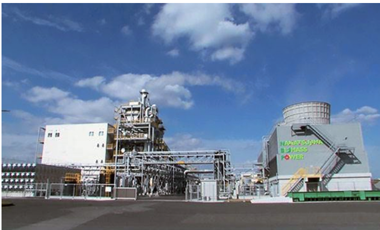
Nanatsujima Biomass Power Plant
