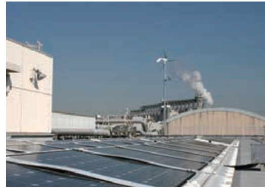
Fig. 4 IHI Corporation Yokohama office photovoltaic generation system
