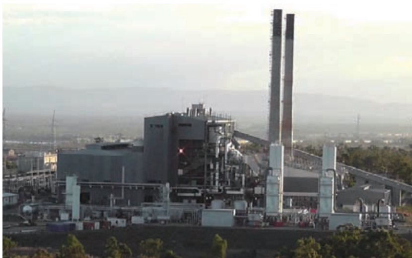
Callide-A power plant with oxyfuel combustion technology
