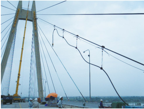
Fig. 22 Removal of stay cable
