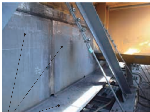
Fig. 19 View of girder after replacement and welding
