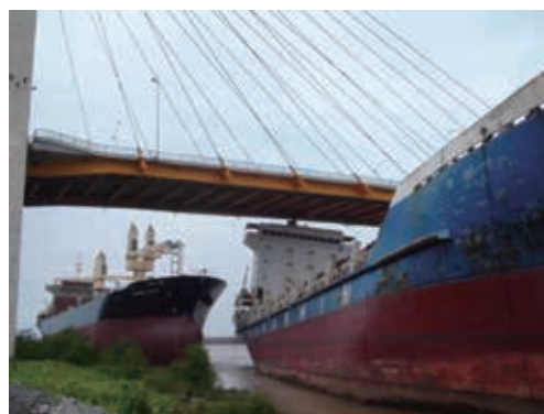
Fig. 2 General view after ship collision
