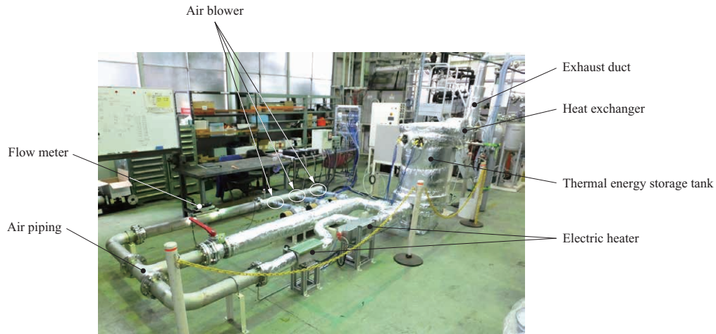
Fig. 3 Picture of packed bed thermal energy storage system
