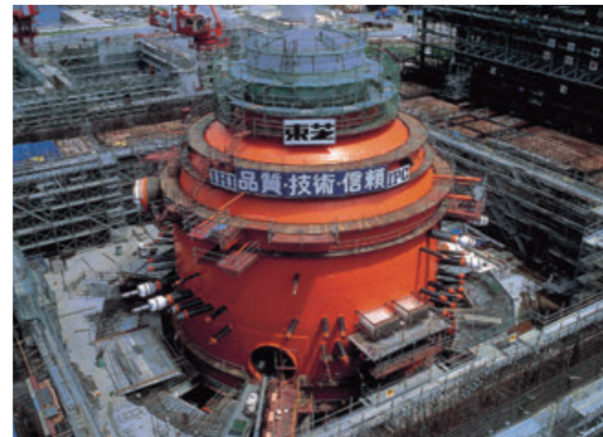
Containment vessel and heavy structures Photo courtesy of Tohoku Electric Power Co., Inc.
