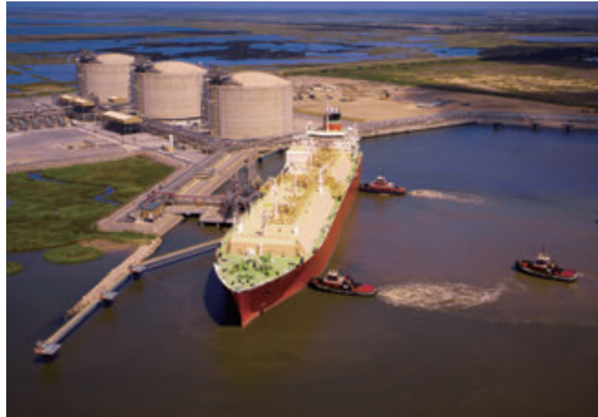
LNG receiving terminal (Semptra's Cameron LNG receiving terminal in Louisiana, USA) Photo courtesy of Semptra LNG ©All rights reserved by Semptra LNG
