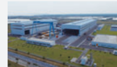
● IHI INFRASTRUCTURE ASIA CO., LTD. (VIETNAM)
