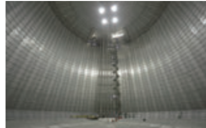
Membrane of world's largest underground LNG tank Photo courtesy of Tokyo Gas Co., Ltd.
