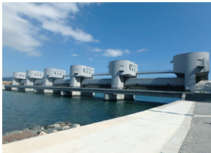
River gate (Kesengawa Gate)
