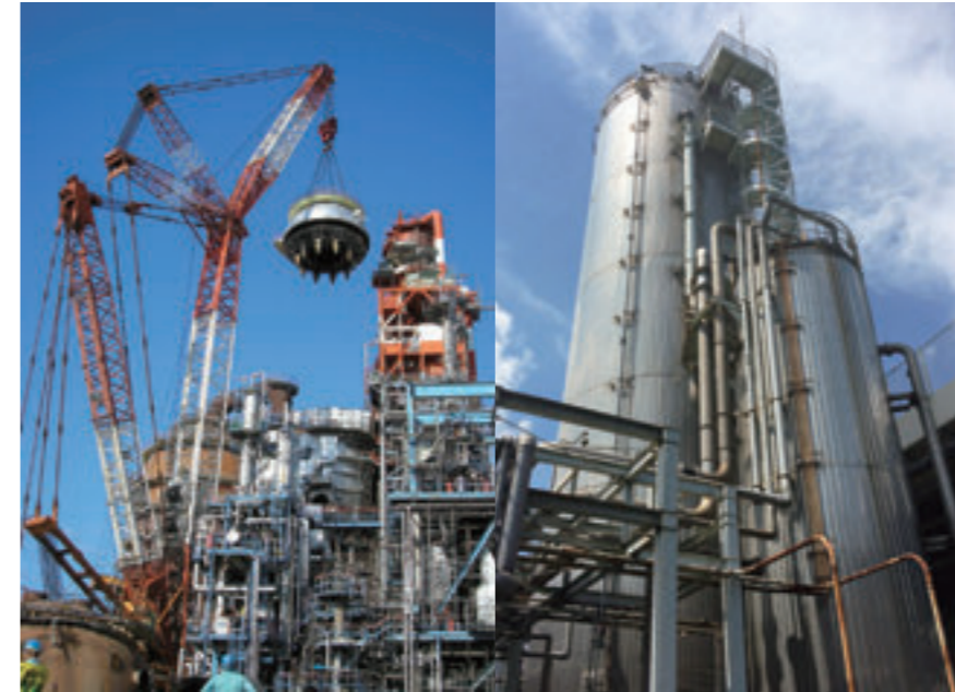
Pressure vessels / Wastewater treatment facility
