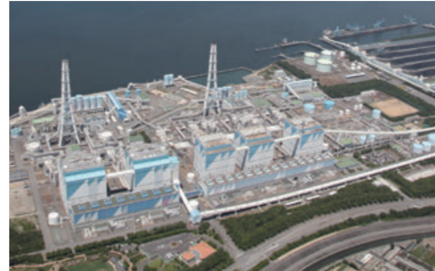
Ammonia combustion technology Photo of Hekinan Thermal Power Station courtesy of JERA Co., Inc.
