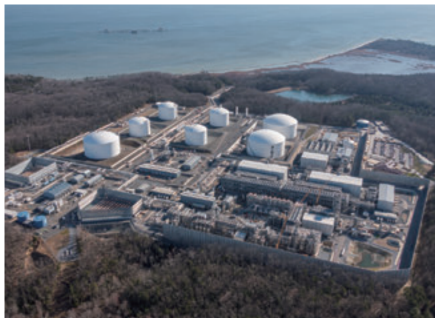
Natural gas liquefaction plants
