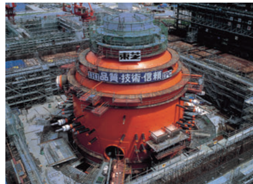
Containment vessel and heavy structures
