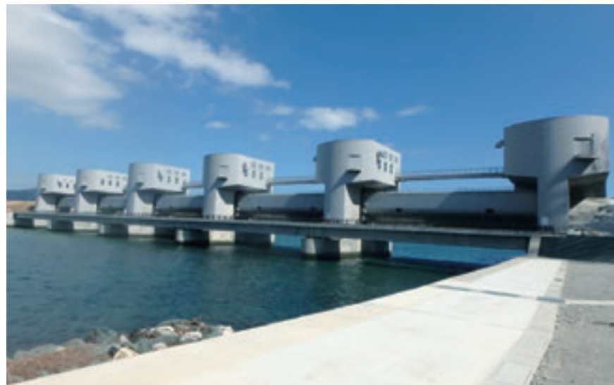
River gate (Kesengawa Gate)
