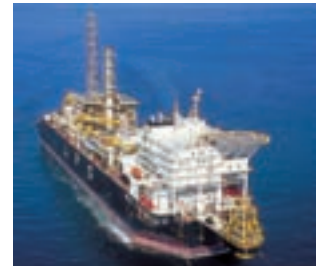
Floating LPG production, storage, and offloading facility
