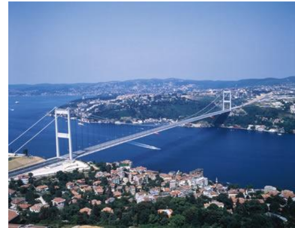
The 2nd Bosphorus Bridge, for which IHI received an order for rehabilitation work
