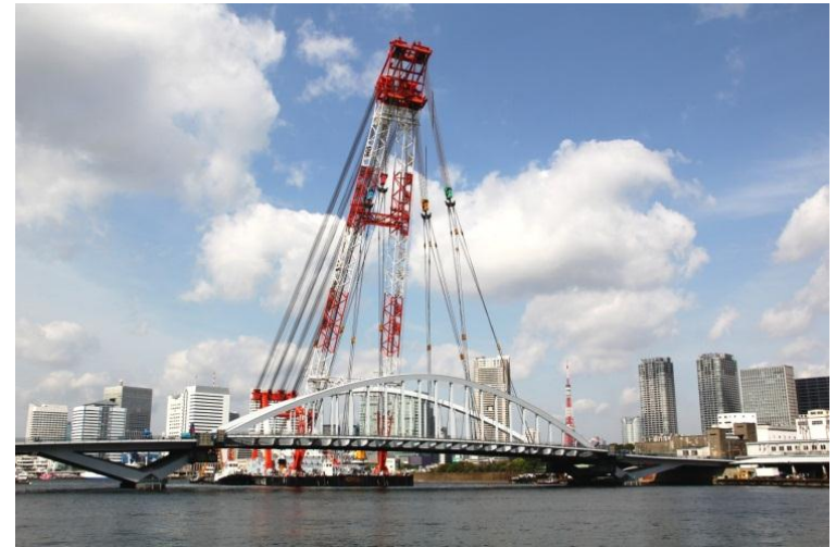
Constructing Tsukiji Bridge
