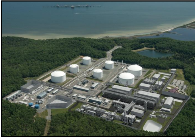
(image of completed project)
