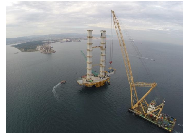
Erecting lower horizontal beam of south tower
