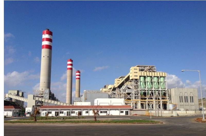
Operating large scale coal fired boiler IHI has completed in Morocco.
