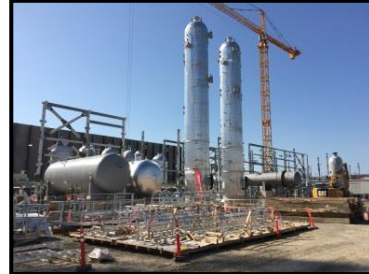
Aerial photo as of Jun 2016 Acid Gas Absorbers installation
