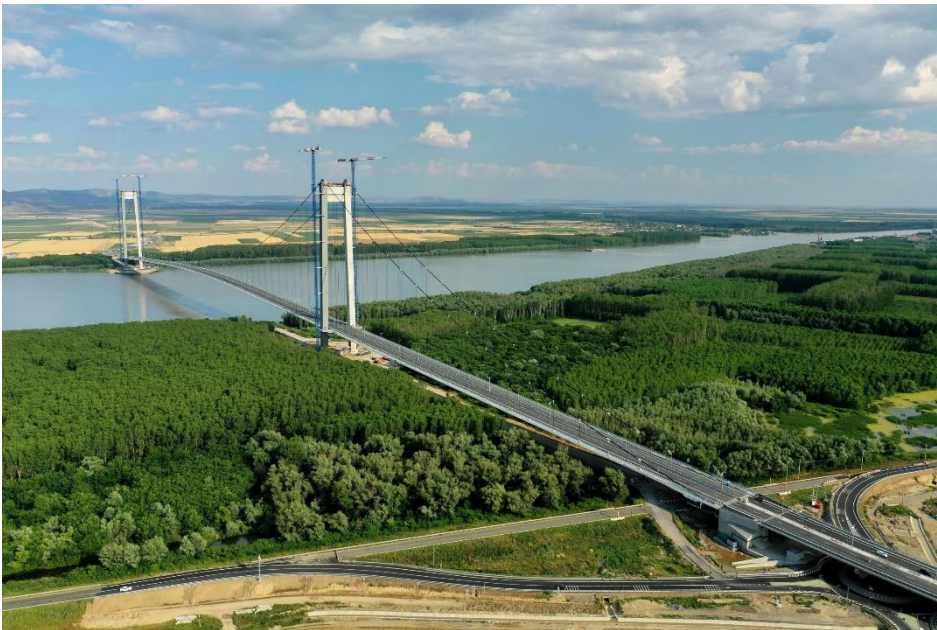
Braila Bridge in Romania
