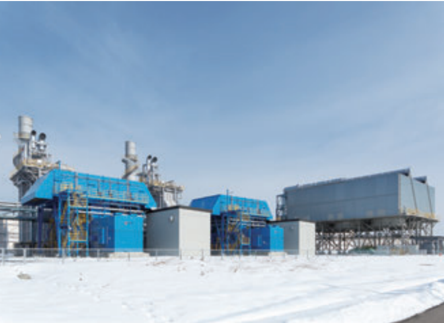
LM6000 gas turbine power plant
