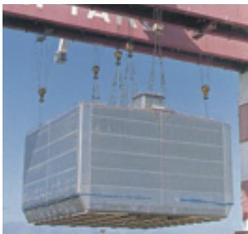
An SPB tank during installation on an LNG carrier
