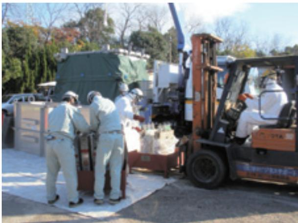
Electrical device using high concentrations of PCBs in transit
