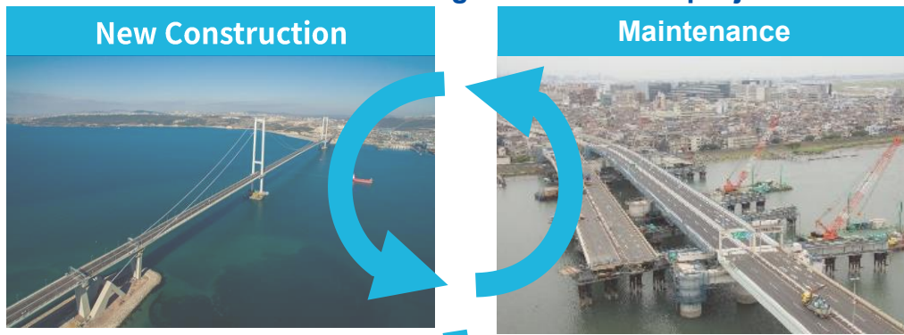
Photo courtesy of Metropolitan Expressway Co., Ltd.
