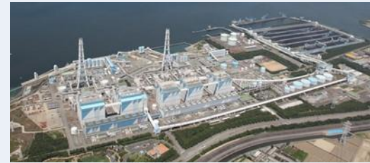
JERA's Hekinan Thermal Power Station
