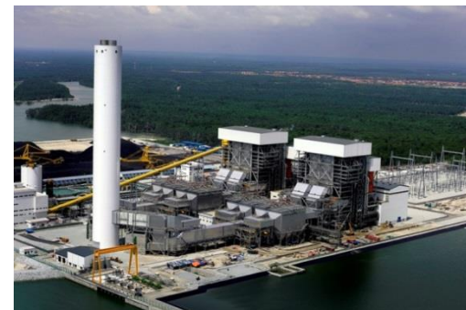
Large, high-efficiency coal-fired power plant
