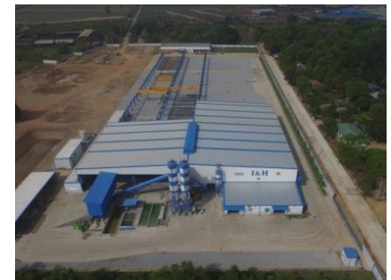
Myanmar concrete products plant opened in April 2017
