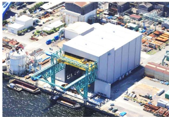
New works for manufacture of steam generators for PWRs (in the Headquarters Representative Office, Yokohama)
