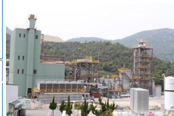
Coal combustion test facility within Aoi Works
