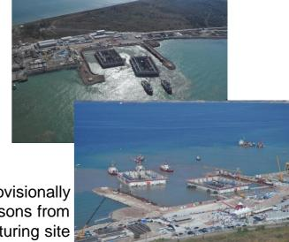
Concrete caissons for the main tower foundation section were provisionally completed in September 2013, and towing these from primary manufacturing site (a makeshift dry dock) to secondary manufacturing site (makeshift wet dock) was carried out. Under the current plan, the building of the caissons at the makeshift wet dock will be completed in March 2014, and sunk and installed under the sea at the north-south main tower location.
