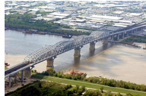
Huey P. Long Bridge, United States (Widening work completed July 2012)
