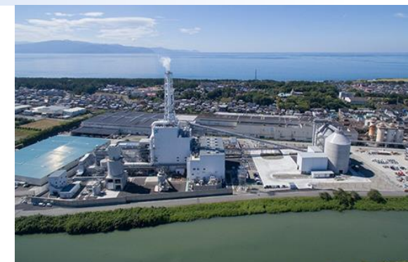
<Thermal power plant (Suzukawa EC)>
