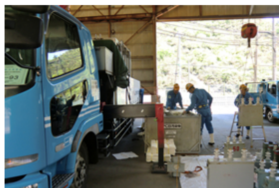
Removal of devices containing PCBs
