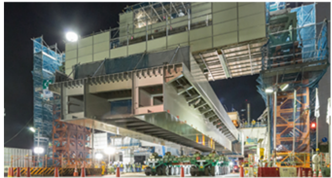
Work site (courtesy of Metropolitan Expressway Company Limited)
