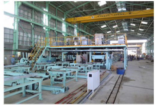
PT Cilegon Fabricators (Indonesia) has installed new panel welders.
