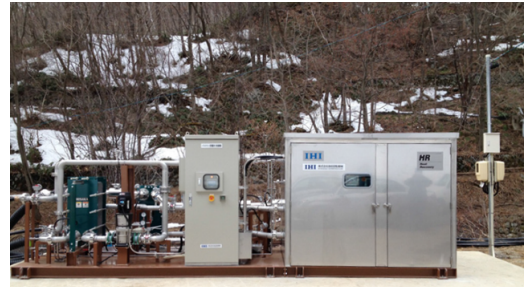
Heat Recovery HR Series: Organic Rankine Cycle Power Generator
