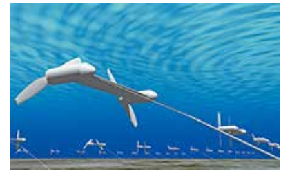
Picture of underwater installation of floating-type ocean current power generation system
