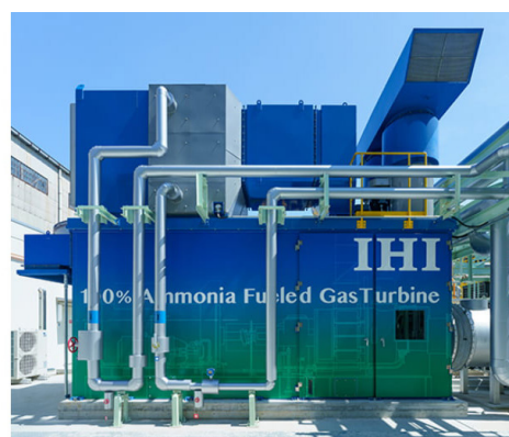
IHI-built IM270 2,000 kW-class gas turbine used in the long-term endurance testing at the Aioi Office
