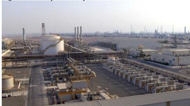
Fig.3 Ammonia production plant in Abu Dhabi
