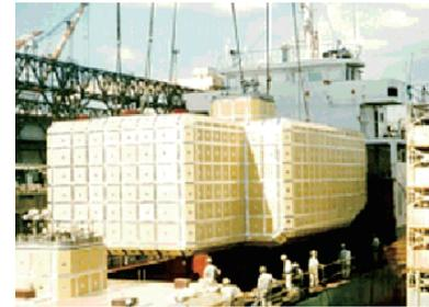
(b) Tank shape for LNG ship
