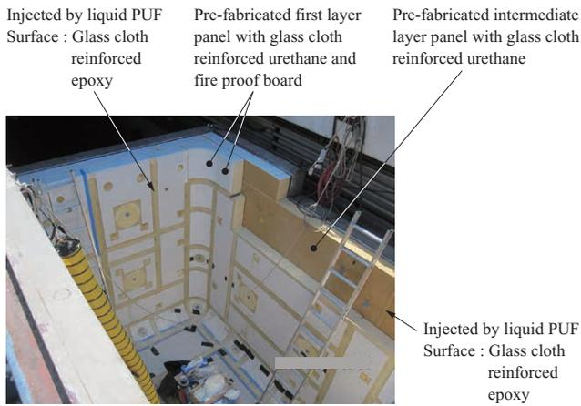
Fig. 6 Insulation panels and secondary barrier work
