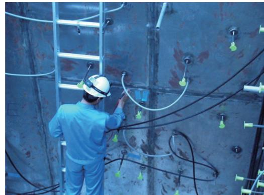
Fig. 8 Helium gas leak test of vapor barrier
