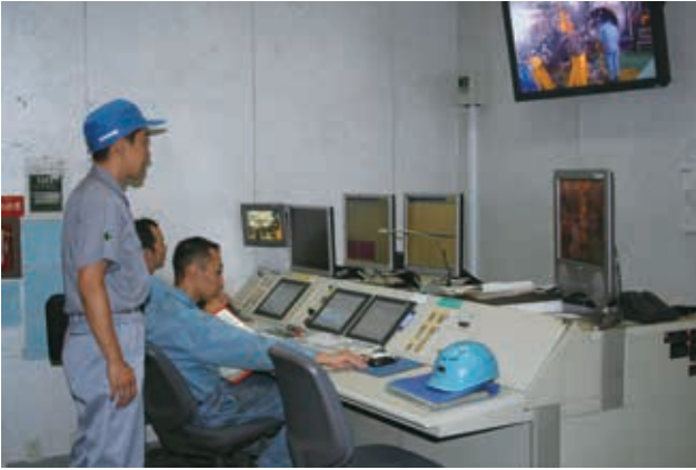
Engine testing control room
