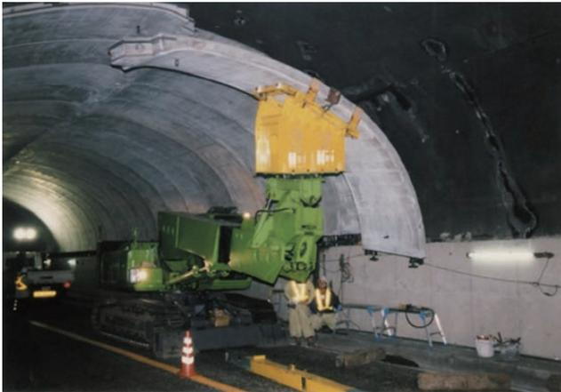
Self-propelled single-purpose machine mode
