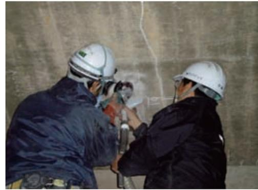
**Fig. 14** Sampling powder from concrete surface
