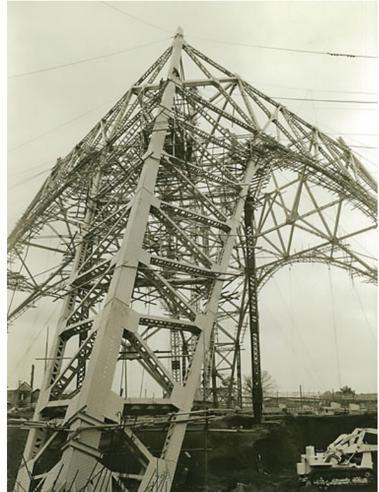
Tokyo Tower under construction (Source : Website of IHI Infrastructure Systems)
