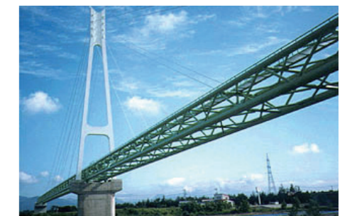
1995 Fukushima Prefecture Niida Aqueduct Bridge (cable-stayed bridge type) (Pipe diameter: 500A x 2 rows, Span: 1198 x 2 m)
