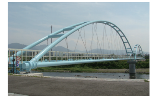
2008 Kagoshima Prefecture Komenotsu Aqueduct Bridge (Basket-handle-shaped, Nielsen system Lohse type) (Pipe diameter: 300A, Span: 59.38 x 2 m)
