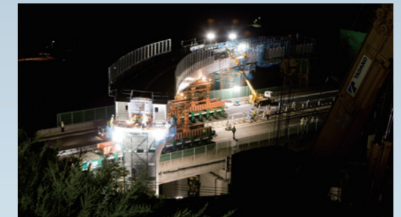
Batch setting of large blocks using a heavy-duty carrier
