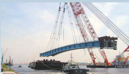
Lifting long girders with a single barge
