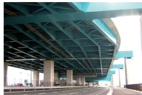
Rakunan Connecting Highway
