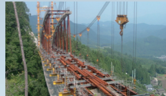
Cable erection method
