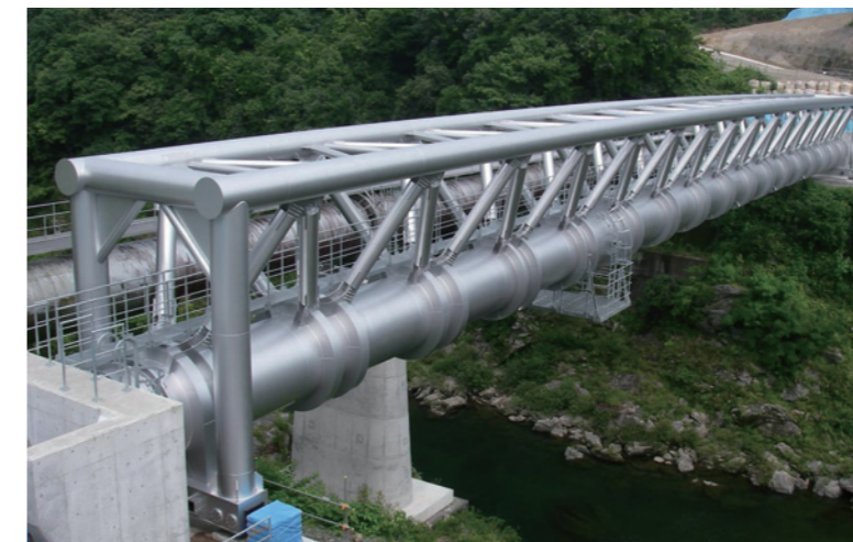
2007 Aichi Prefecture Toyokawa Aqueduct Bridge (inverse trigonometric stiffening truss type) (Pipe diameter: 2,000 mm, Span: 73.6 m)
