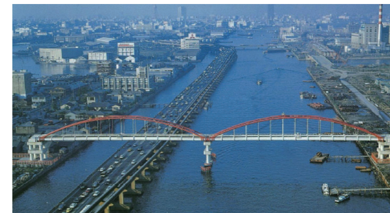
1967 Tokyo Ooi No2 Aqueduct Bridge (Langer stiffening type) (Pipe diameter: 1022A x 2 rows, Span: 79.8 x 2 m)
