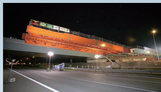
Fast launching erection over heavy traffic
