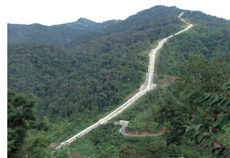
Dainin hydraulic power plant
