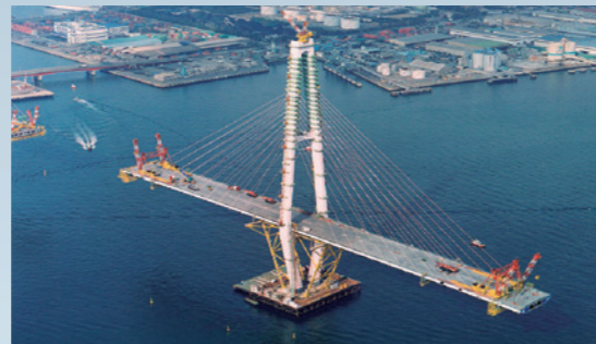
Overhanging erections for cable stayed bridges
